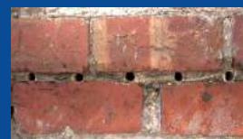
Mortar & bricks saturated with DPC Cream
