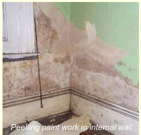
Rising damp shown in internal walls
