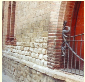
Rising damp in stone wall
