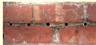
Mortar & bricks saturated with DPC Cream
