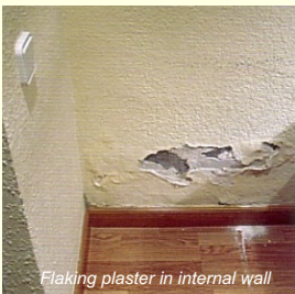
Rising damp shown in internal walls
