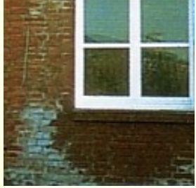
Rising damp in brick wall
