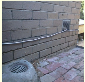
Rising damp in brick veneer wall below damp course
