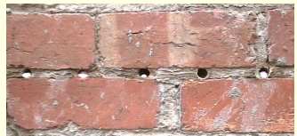
DPC Cream starts penetration
