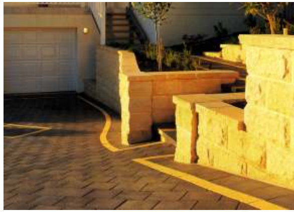
▶ Structural retaining wall
